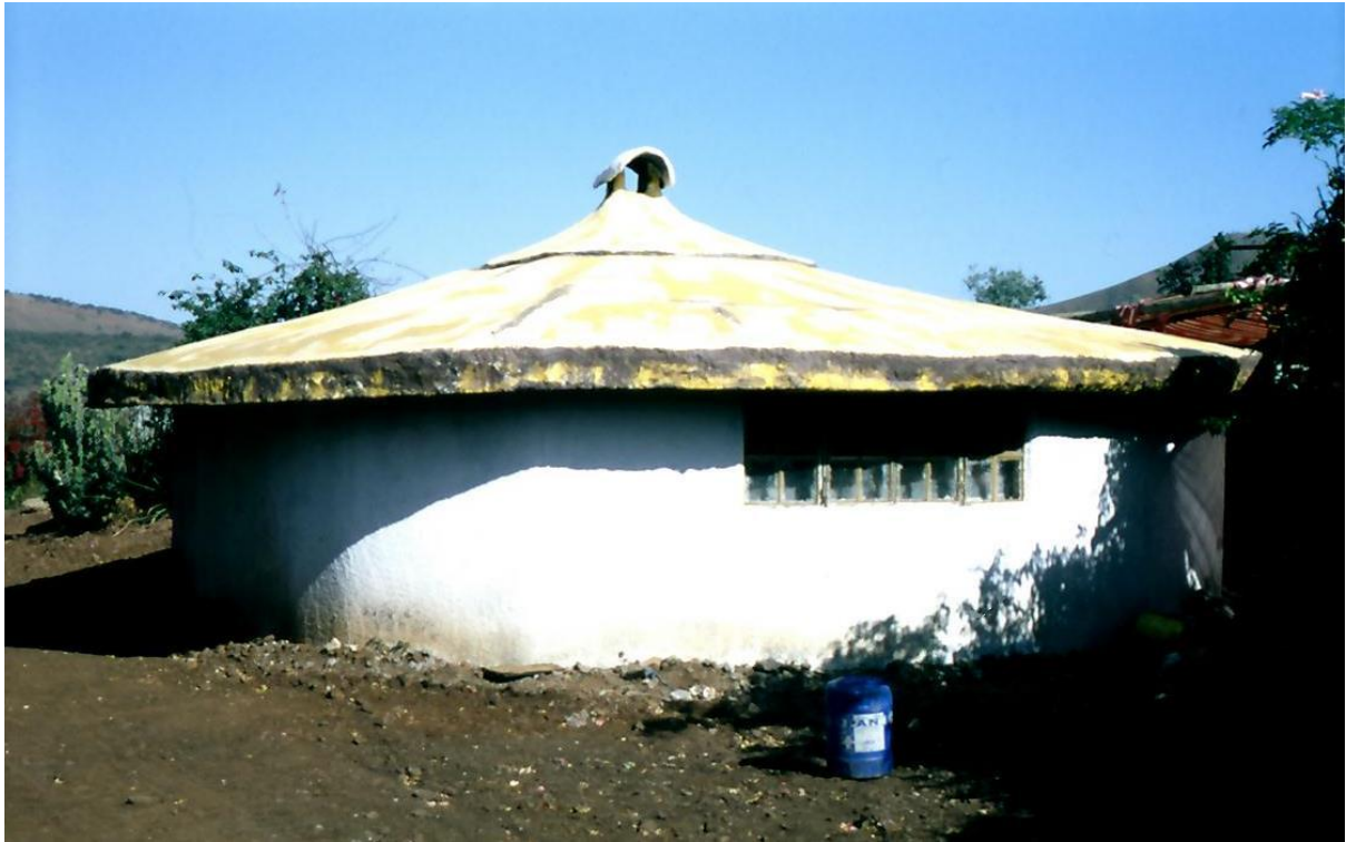
Lucas SITHOLE's studio at Spekboom – supported by carved beams - 1993
